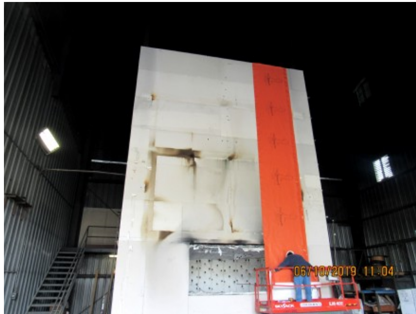
Photo No. 1 Application of Weather Barrier
