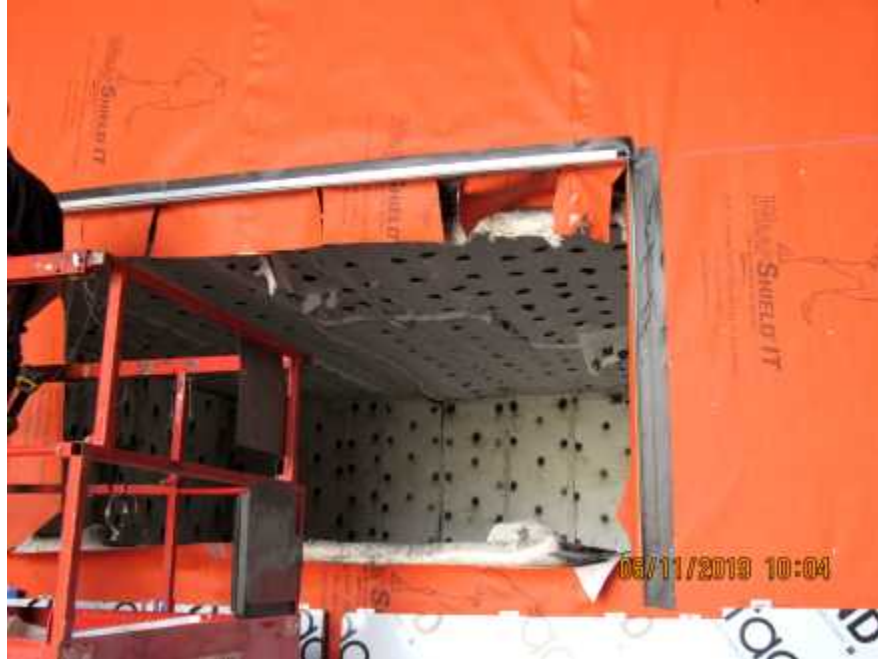
Photo No. 5 Installation of J-Trim around Opening
